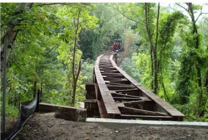
The Salmon Brook Bridge stripped of old decking and ready for new construction in the first week of September.
